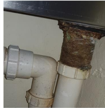
M103: Urinal waste pipes corroded.
