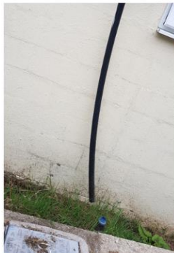
M105: Pipes not secured, disconnected.
