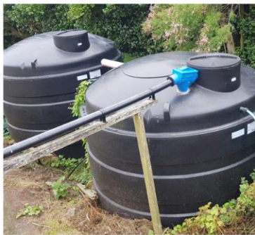
M104: Rainwater harvesting tanks.
