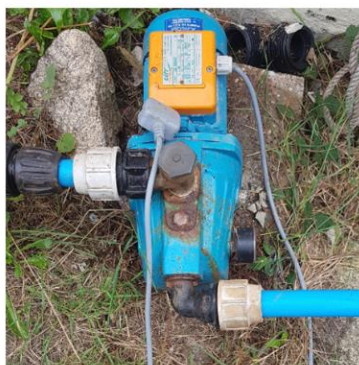
M105: Pipes not secured, disconnected.
