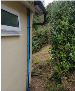
M101: Water inlet pipes.
