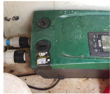
M106: Booster pump, constantly running.
