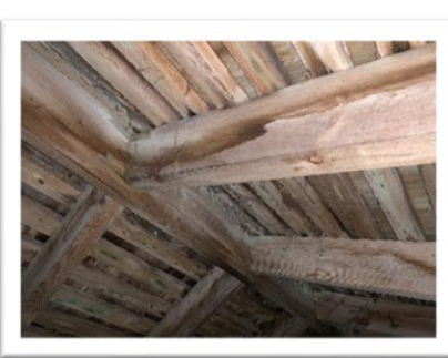
B108: Timber rafters are showing signs of active woodworm and damp
