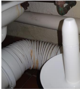
M102: Flex waste pipe + 90 degrees turn. Replace
